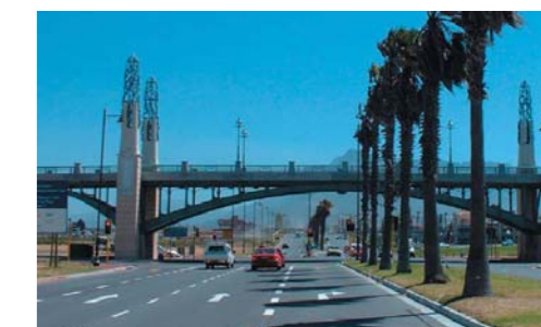
Century City Viaduct, Cape Town
